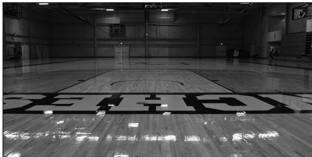
PLAY BALL The newly repaired basketball court floor is now gleaming and ready for action. After ripples began forming on the original court, the floor needed to be updated during a six-week long process this summer.
