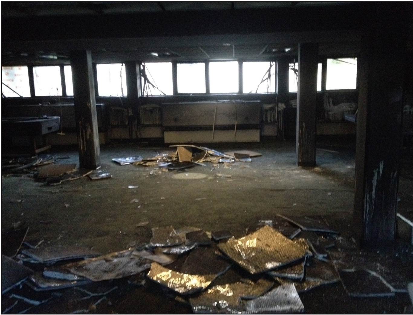
THE AFTERMATH There was a small fire in the basement lobby of Schwalm Hall on Saturday, Sept. 20. The North Manchester Fire Department responded very quickly and was assisted by several other local fire departments. Residents were not allowed to return to their rooms for the night; however, the Red Cross delivered cots and blankets to the Helman Hall and Oakwood Hall great rooms for the displaced students. The residence hall re-opened at 3:30 p.m. on Sunday, Sept. 21. The cause of it is still unknown and the case is under investigation.
