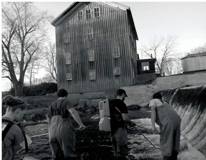
Students construct fish ladder by the Stockdale Dam in Roann, Indiana.
